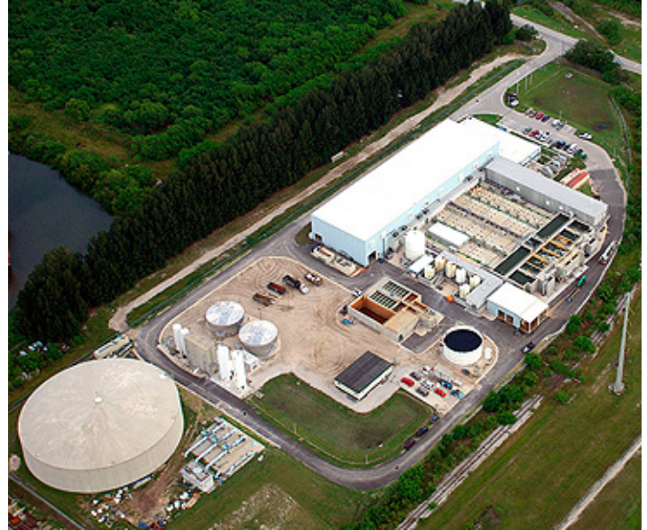
Tampa Bay Water Desal Plant – The first large-scale SWRO in the US
